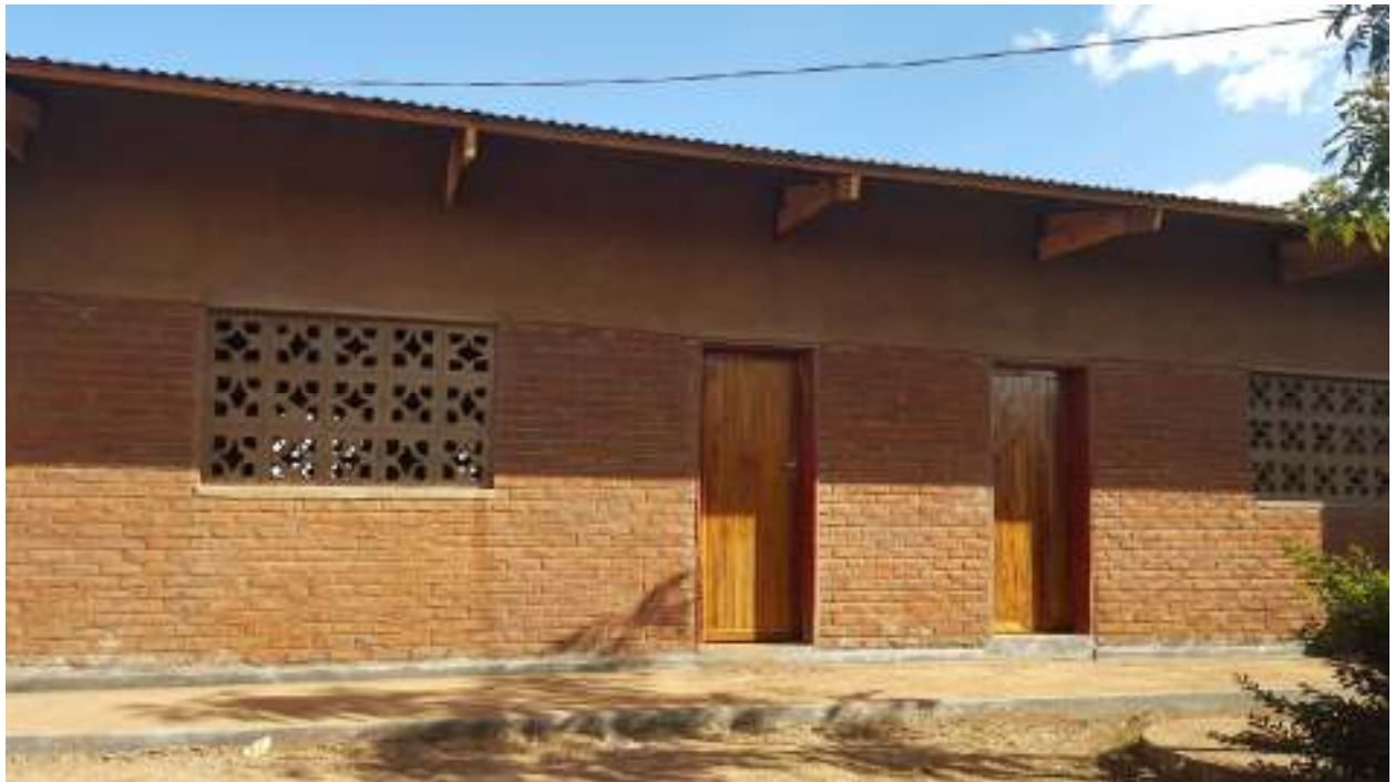
One complete block, painting and fixing black boards remaining
